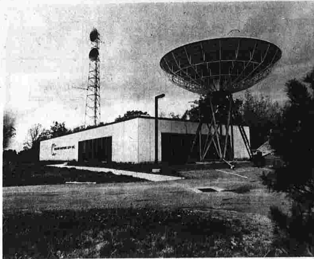
'Earth station' installed
